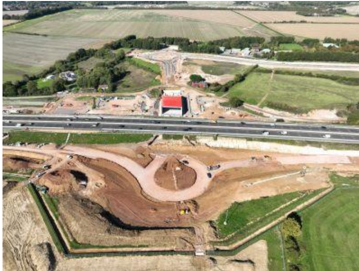
Aerial view of the completed box structure
